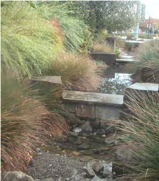
Fig A.6.S12.a: On-site rain garden manages stormwater.
