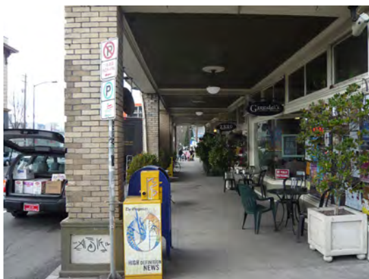
Fig. B.1.S5: Colonnade with sufficient height to allow for light to enter the space.
