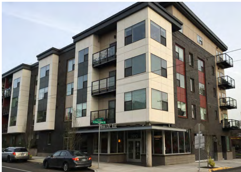
Fig. B.4.S8.b: Building base established through a change in materials and depth and building top established through a prominent cornice line.
