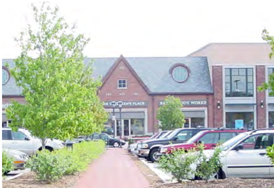
Fig. A.3.S3.a: Pedestrian walk through parking area.
