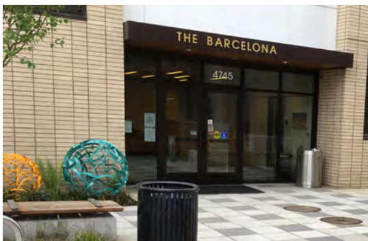
Fig. B.6.S4: Canopy sign which does not project beyond the face of the canopy upon which it is attached.
