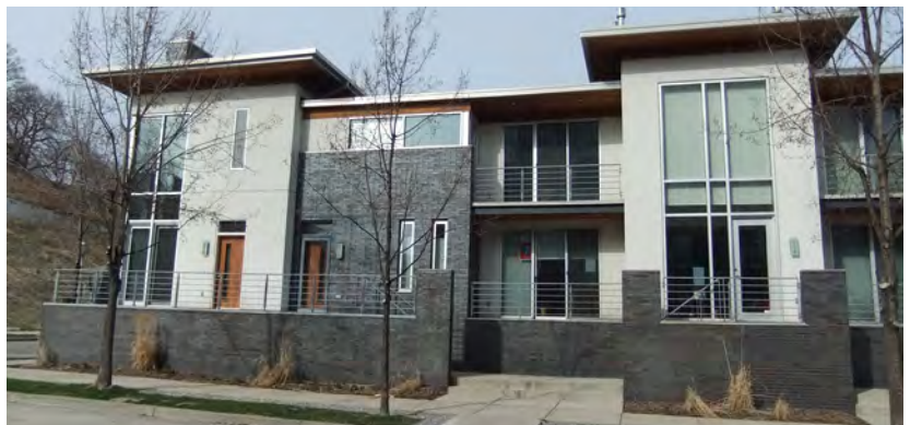
Fig. B.1.S2: Variation in building height help reduce the volume of a facade longer than 30 ft. in length.
