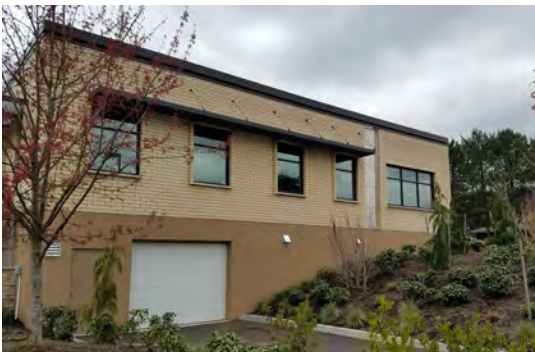
Fig. A.4.S7.a: Loading area is integrated into the rear of the building.
