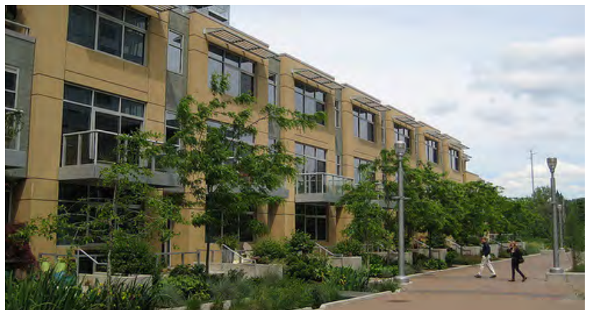
Fig. B.4.S15.b: Townhouses with facade offsets, alternating finish patterns, projecting balconies, and recessed entries.
