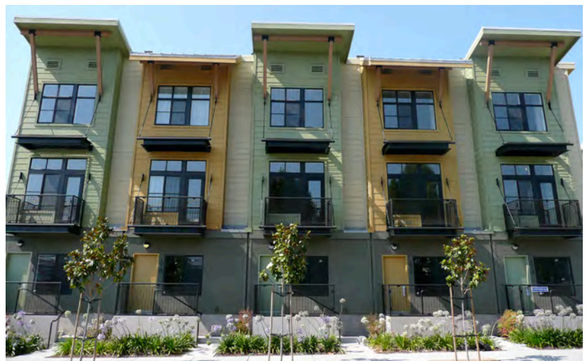
Fig. B.3.S8: Ground-floor units providing individual entries accessed directly from the street.
