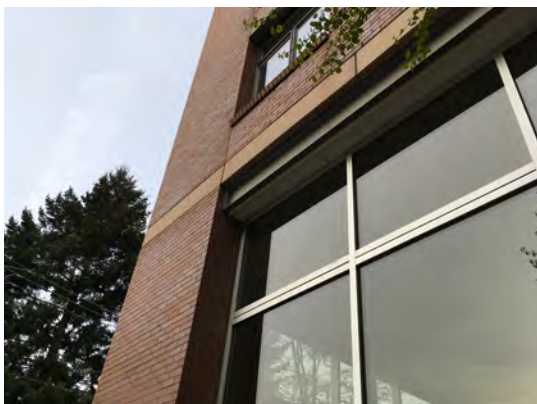
Fig. B.5.S5: Recessed windows provide a sense of depth and shadowing on the facade.
