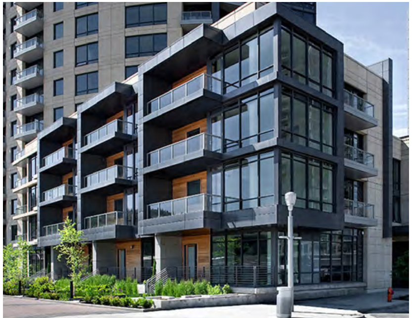
Fig. B.8.S1.c: Finished wood, finished metal, and glass are used as primary materials.
