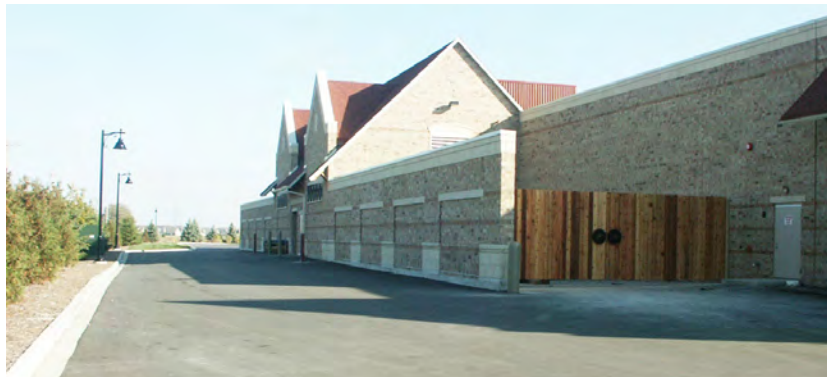
Fig. A.4.S7.b: Loading area at the rear of the building, visually screened by a wall matching the building architecture and by landscaping at the property line.
