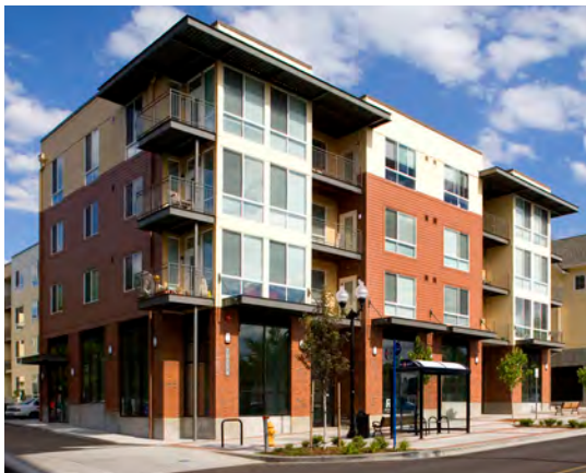
Fig. A.2.S2.a: Corner building located with frontage along both streets and oriented to the street with higher functional class.
