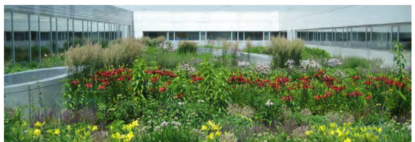
Fig B.2.S2.a (right): Green roof treatment limits solar reflectance on a flat roof surface.
