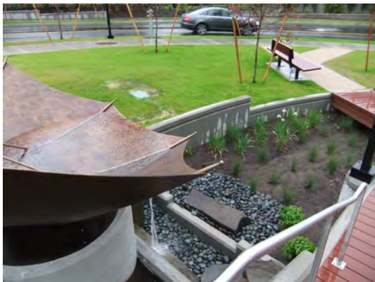
Fig. A.5.S3.a: Art feature collects rainwater for use in open space landscaping.
