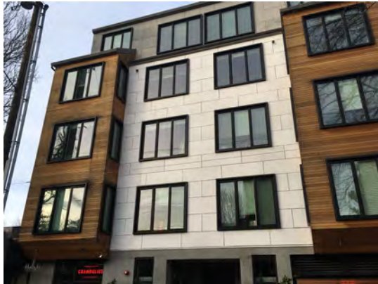
Fig. B.8.S1.a: Finished wood, glass, and fiber reinforced cement siding panels are used as primary materials on this multifamily building.
