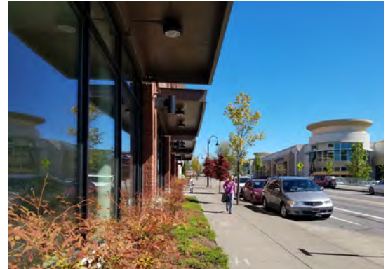
Fig. B.2 Existing Civic Drive improvements with a commercial frontage and planter.
