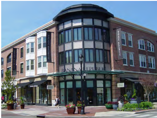
Fig. B.3.S6.a: Corner entry provides awning for weather protection and enhanced paving.
