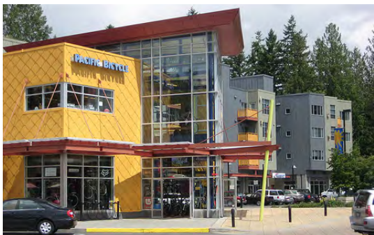
Fig. B.3.S6.c: Commercial entry provides a change in building form and enhanced transparency.
