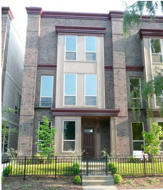
Fig. B.4.S13.a: Ground floor residential entries transition from the street through an increased setback and raised first-floor elevation.
