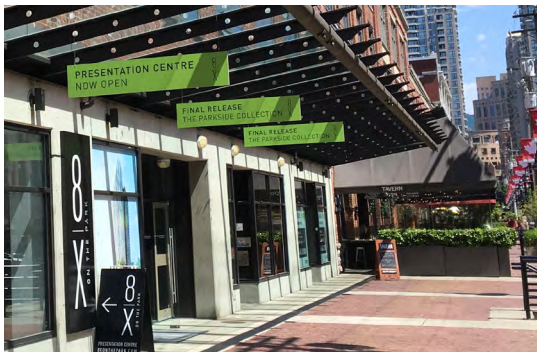
Fig. B.6.S2: Under Marquee signs hanging from a canopy maintain an 8-ft. clearance above the sidewalk.
