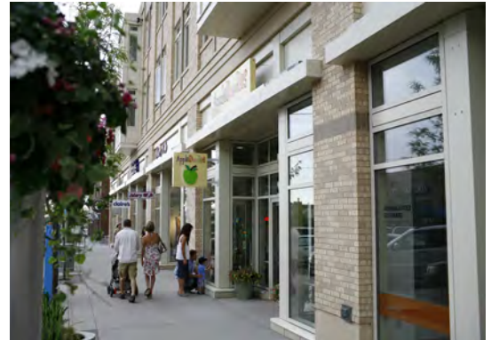
Fig. A.2.S1.a: Building frontage should reinforce the urban character of the neighborhood.
