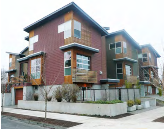
Fig. B.4.S14: Townhouse style building facade treatments wrapping the building corner and continuing across multiple building facades.
