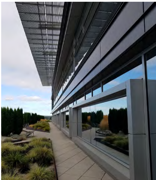
Fig. B.4.S7.b: Building with long axis oriented east and west with unobstructed solar access to the south wall.
