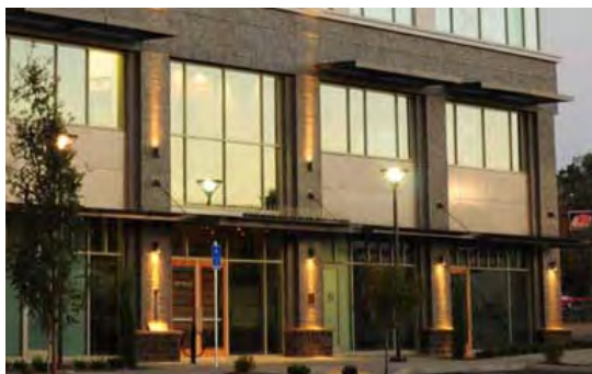
Fig. B.4.S9.a: Ground level facade incorporating pedestrian scaled detailing including awnings and wall-mounted lighting fixtures.
