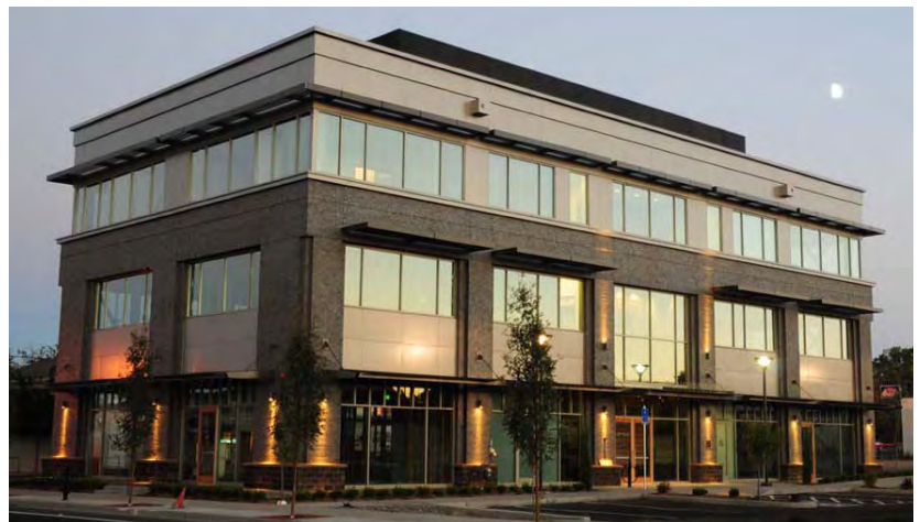
Fig. B.2.S2.d: Flat roof with parapet capped with cornice details.
