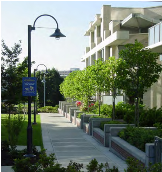
Fig. A.7.S2.a: Cut-off pole light used to illuminate an internal pedestrian path and shared open space.
