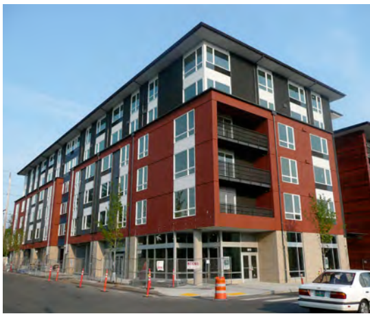
Fig. B.1.S2.a: Individual wall plane height does not exceed 4 stories before horizontal articulation is provided.
