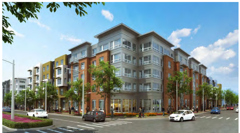
Fig. B.5.S14: Multifamily building providing high levels of transparency facing adjacent streets.
