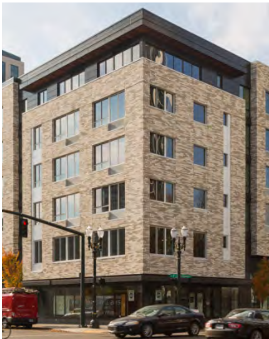
Fig. B.1.S2.b: High levels of transparency on the top floor facade help minimize perceived building height.
