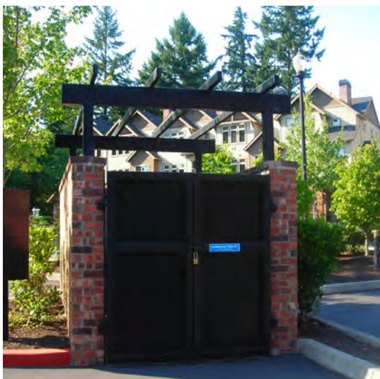
Fig. A.4.S8: Collection area screening enclosure using high quality materials similar to the primary structure.
