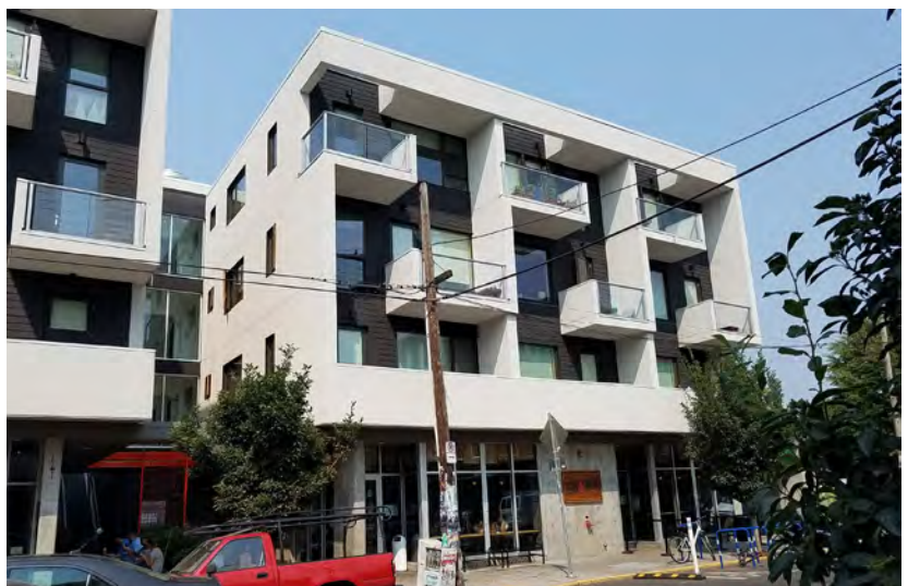
Fig. B.1.S6: Significant massing change over 10 ft. in depth provided to break up massing on long building facade.
