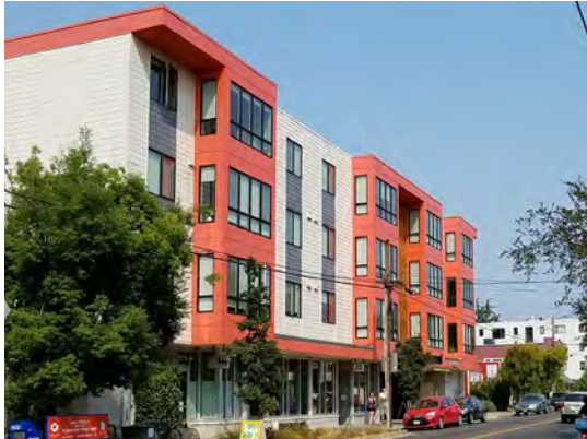
Fig. B.4.S10: Facade rhythm established through a series of vertical reveals between building masses.
