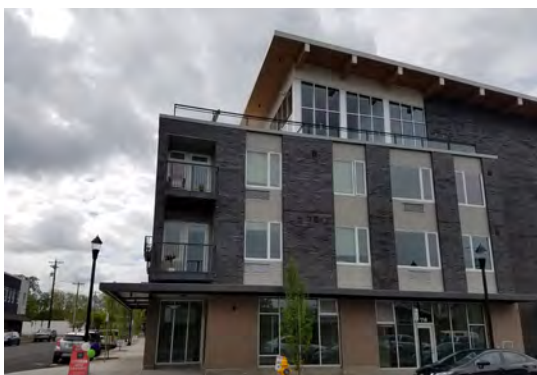
Fig. B.1.S1.a: Articulated wall planes break down building massing to reflect a human scale.
