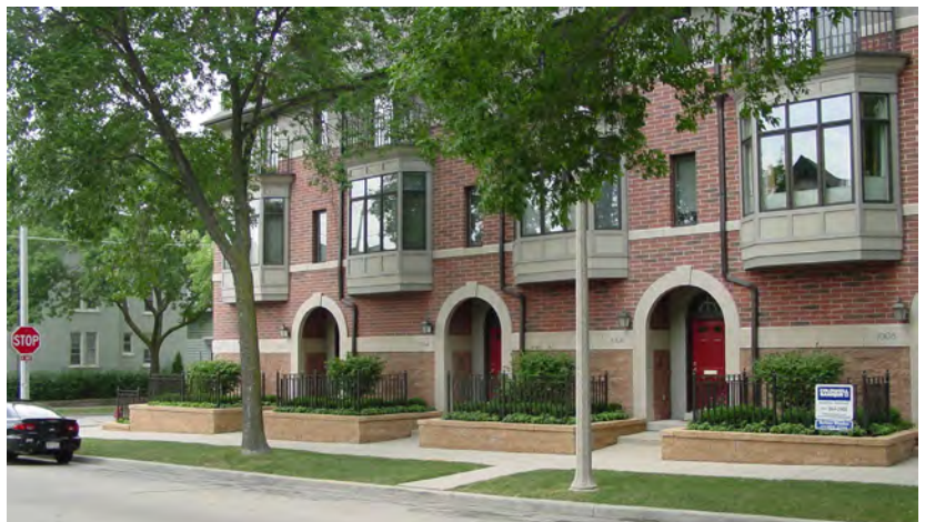
Fig. B.4.S13.b: Ground floor residential entries transition from the street with a landscape planter and recessed door.
