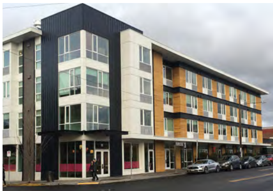
Fig. B.4.G2: Through-wall mechanical units are flush with the facade and integrated into the facade design to minimize their visibility.
