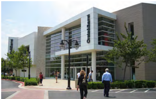
Fig. B.3.S6.b: Primary commercial entry provides a change in building form and enhanced transparency.
