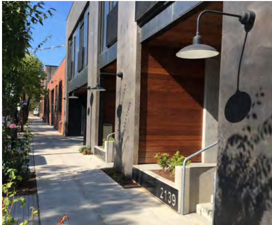
Fig. B.3.S9.c: Recessed individual unit entries are separated from the street with landscape planters and steps up to the door.
