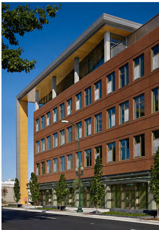
Fig. B.4.S8.a: Building base established through a change in materials and top established through a projecting roof line.
