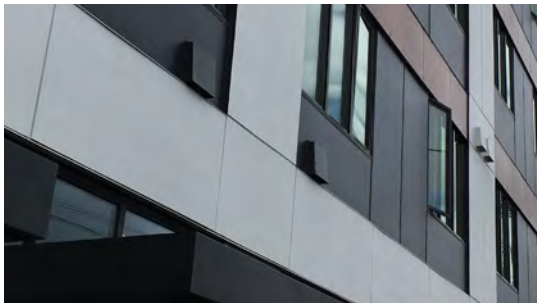
Fig. B.4.S3: Vent covers utilize similar materials and colors as the surrounding facade area to minimize their appearance.
