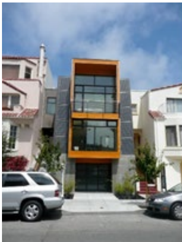
Integrated solar wall panels on a townhouse.
