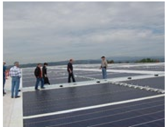
Flat roof solar film on an industrial building.
