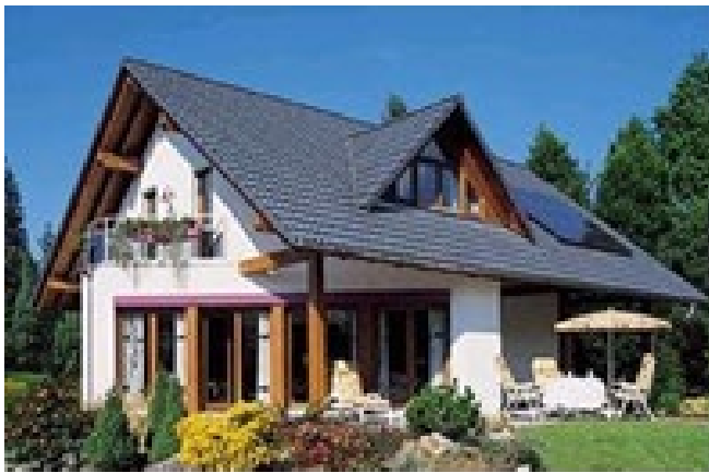
Roof-top solar panels on a single-family residence.
