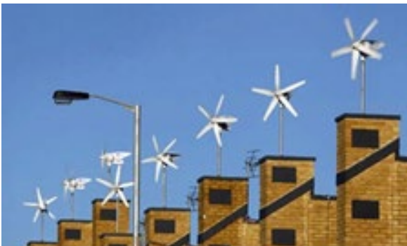
Small-scale wind turbines mounted on a roof.
