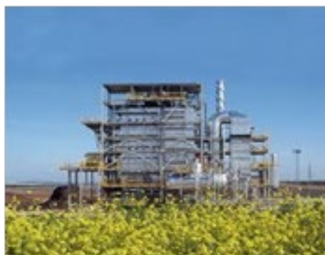
Biomass Plant From: Gestamp
