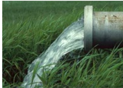
In-Outfall Pipe Micro-Hydro System
