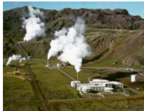
Geothermal Energy Generation Facility Plant
