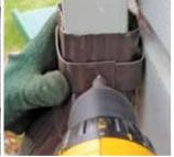
Wiggle the attached downspout assembly to make sure it is secure.
