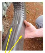
Place screws only on the top or side of the gutter.
