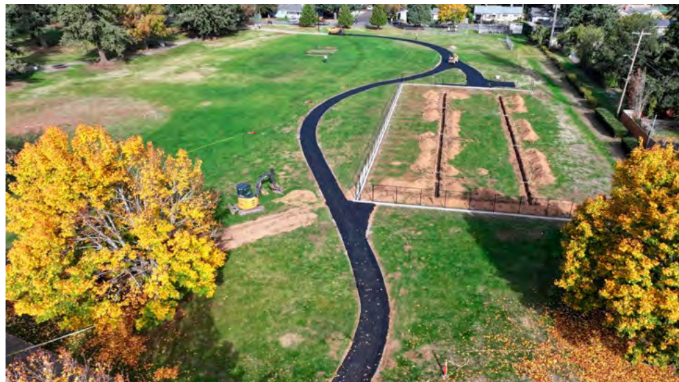
Rockwood Central Park construction on new accessible pathways and community garden.
