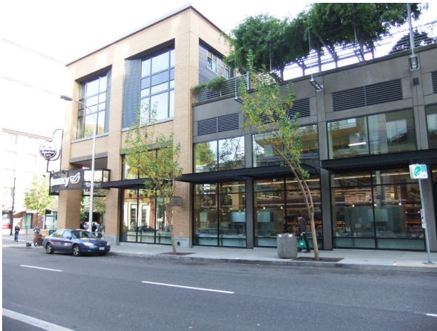
Figure 4.1152(B)(1)(S4). Larger buildings include multiple masses to break up the façade.
