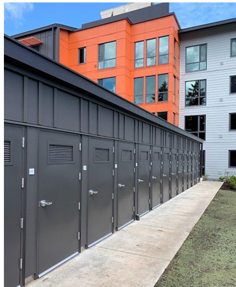
Figure 4.1152(A)(4)(S8). A central storage facility on the exterior of the building.
