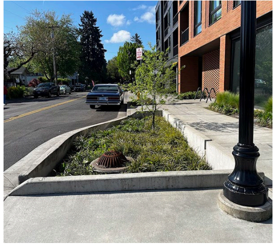
Figure 4.1142(F)(1). Rain garden located in a bulb out.
