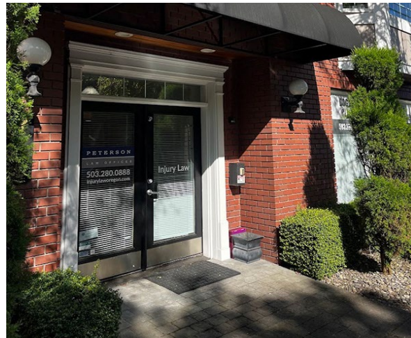
Figure 4.1152(A)(7)(S3). Light fixtures around an entry include vandalism and weather-resistant covers.
