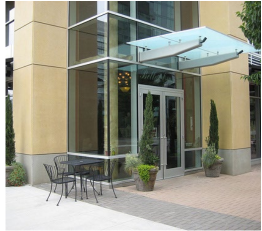
Figure 4.1152(B)(3). Entries are highlighted, adding character and providing wayfinding.
