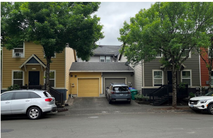
Figure 4.1152(A)(4)(S9). Garage doors on townhouse units match the main building's color and trim.
