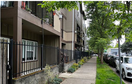
Figure 4.1152(A)(5)(S8). Townhouse-style units are provided open space with balconies and patios.
